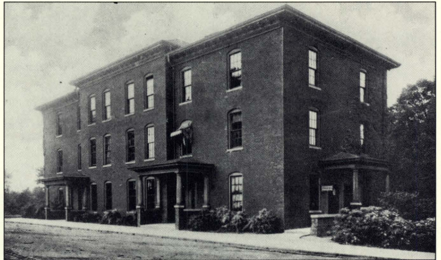
South College, one of the College's homes on "the hill" during the School's first quarter century.
